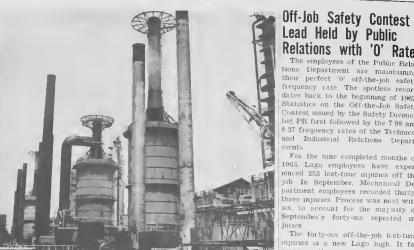
THE SKYLINE is being lowered figuratively speaking. Shown are addition and a shortened stack, which no longer serves as an exhaust, but directs heat into the duct work leading into the added section and new stack. E. LINJA di horizonte ta wordi habri, pasando sa un manera figurativa. Combination Units 6 & 7 ta parce riba e perfil. No tin un sucesor pa transferi calor di parti pafor, y un chimenea mas cortico cu lo bai sarti mas cu un apertura e trape.
